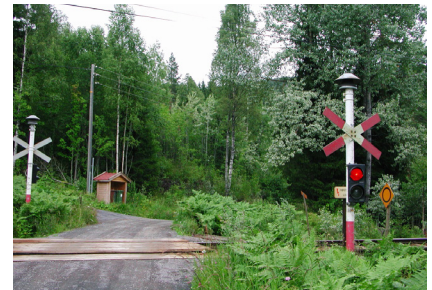
Vegsignalanlegg / Warning lights
