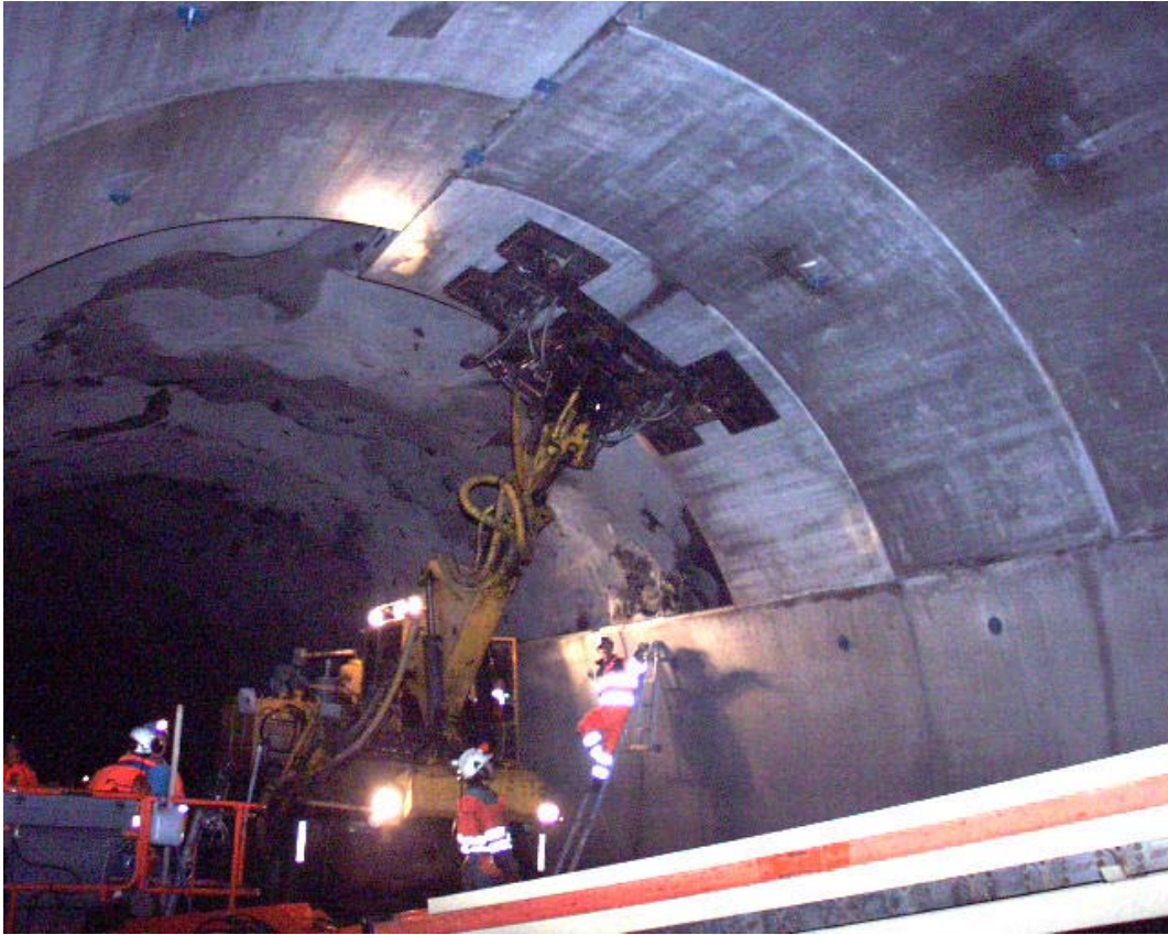
Figur 15: Betong elementhvelv under montering
