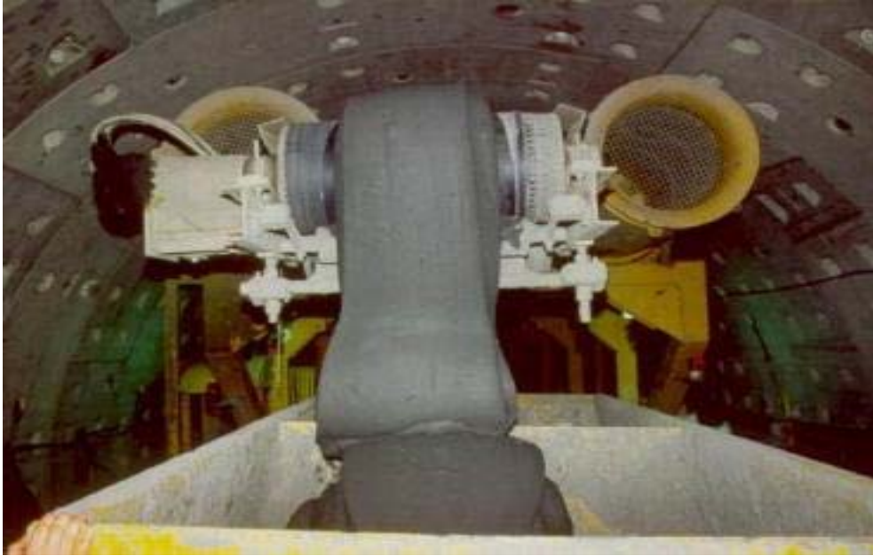
Figure 20: Ideal consistency of the conditioned material using EPB
