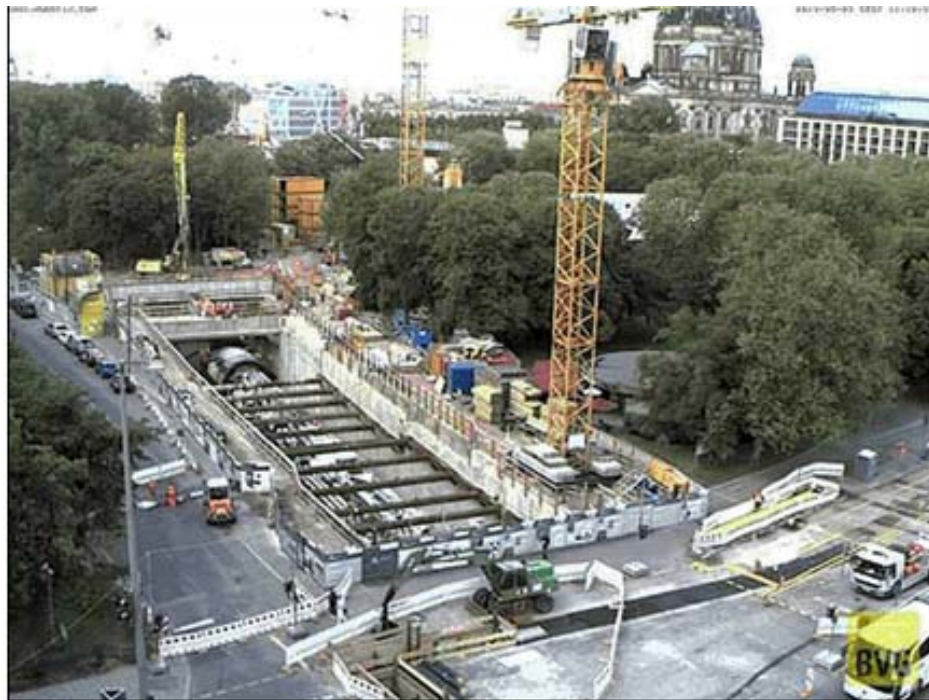
Figure 33: Rig area U5 Metro project in Berlin (Amberg archive)
