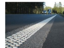
Profilert vegoppmerking nedfrest plant spor
